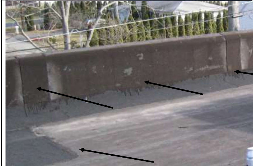
Photo # 27- Patching along north wall
