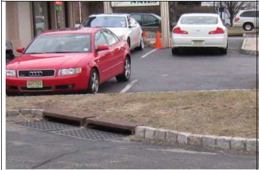
Photo # 2- Parking lot drains along the Belgian block curbing south west corner.
