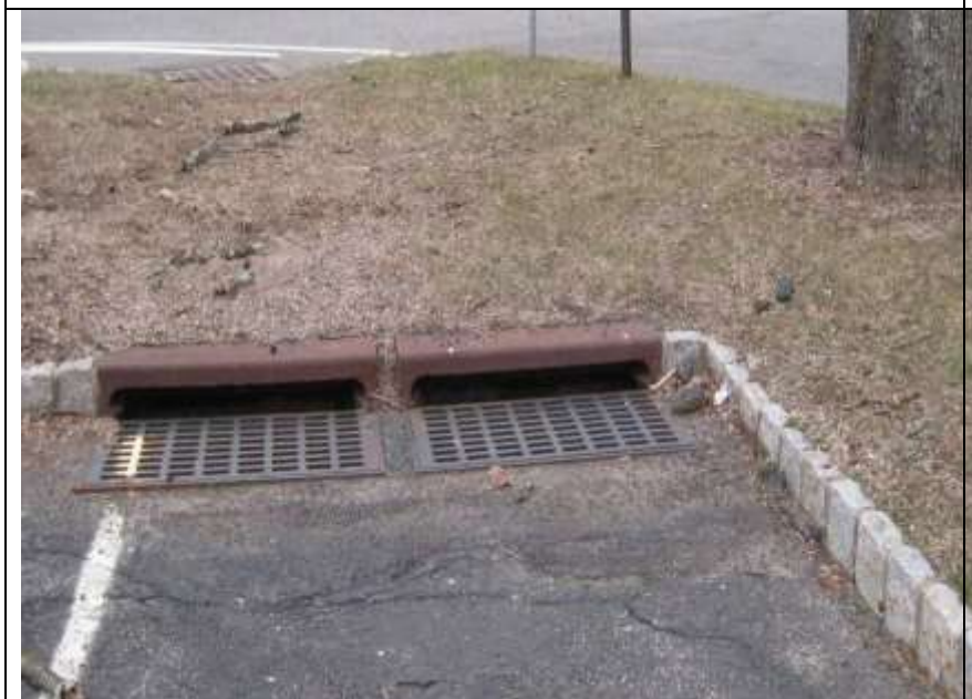
Photo # 3- Parking drains along north west corner at Commercial Road and Park Place.
