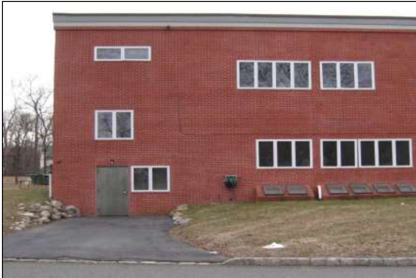
Photo # 7- (Topology)- North east left corner of building. Drainage toward rear metal door that shows rust and corrosion.
